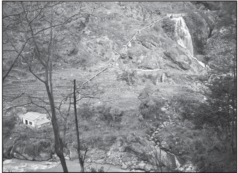
A typical, small hydro-electric plant, sitting at the base of some big waterfalls.
