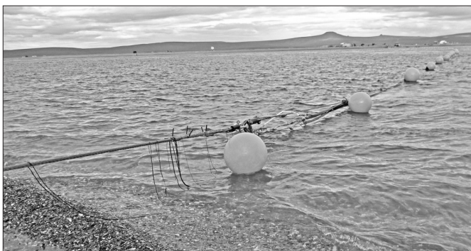
The cable reached the Teller beach after slowly being pulled across the channel.
