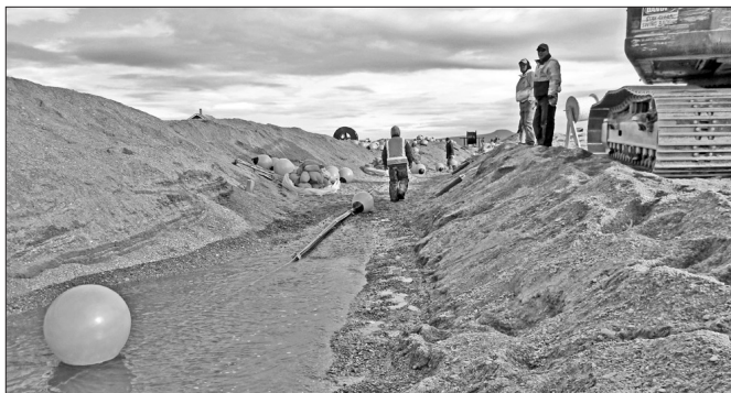
The Brevig Mission trench at the start of the cable pull.
