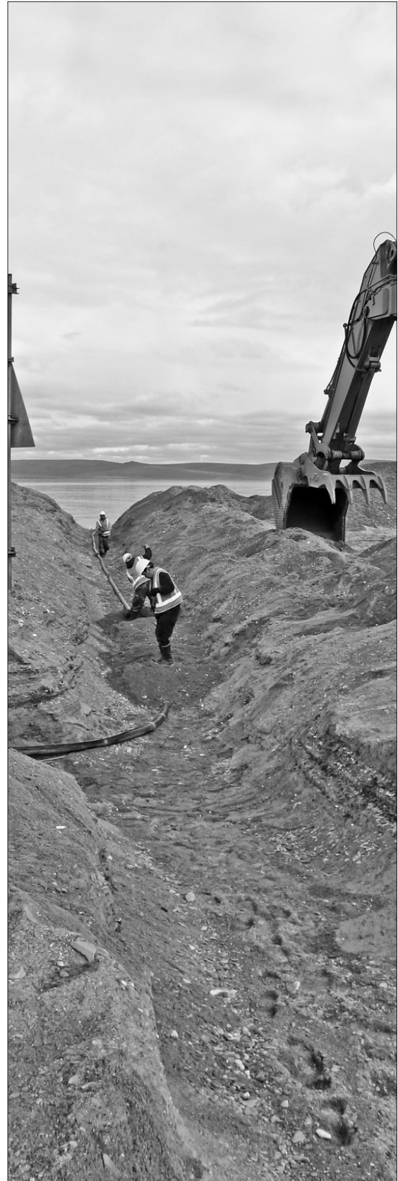
Starting to backfill the primary trench in Teller.
