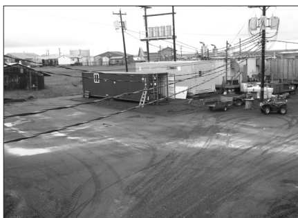
The finished installation of the control module and storage module.
