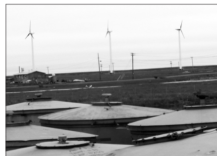
These three Northwind 100 kW wind turbines should be fully operational in 2011.
