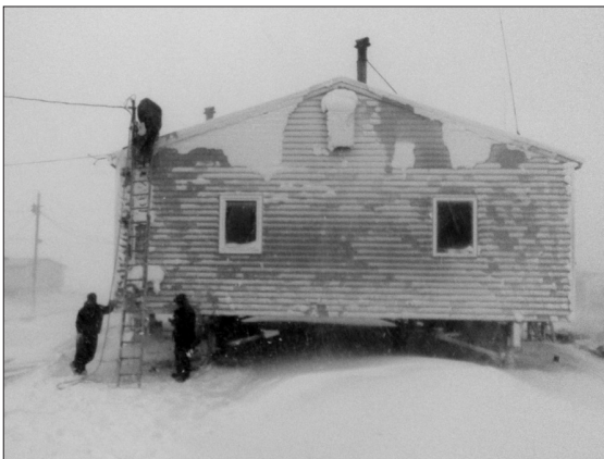
Linemen Matt Kruger and Brian Gundvaldson and plant operator Stuart Kingeekuk worked in blizzard conditions to restore power.
