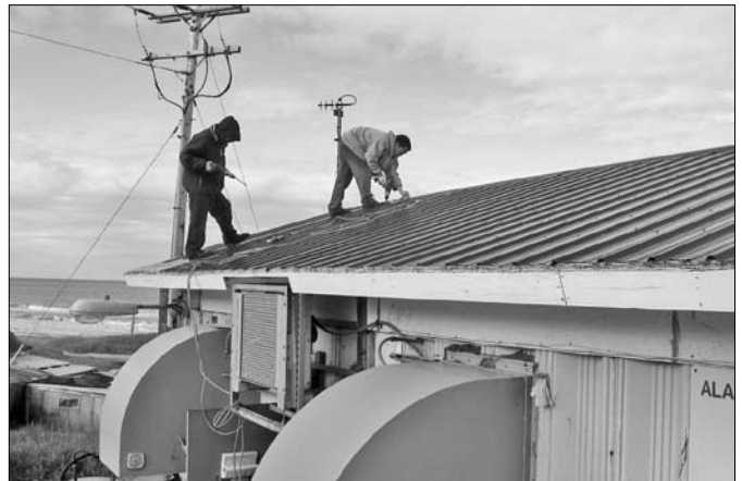
New plywood, tin sheeting and fascia was installed on the roof and all the seams and screw holes were caulked to prevent leaking.
