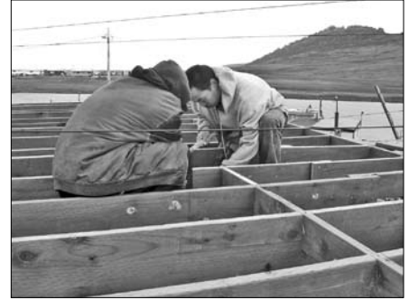
Building trusses for the roof.
