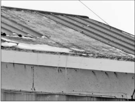
The old, decrepit roof was full of holes that allowed water to leak into the plant.
