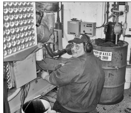
Operator Bill Crisci performs an engine oil change.
