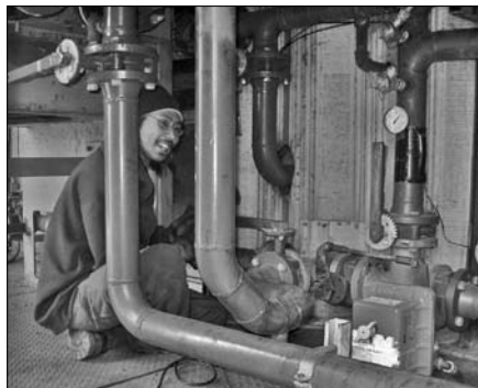
Above: Greg Oxereok preps the piping and removes rust prior to repainting (left).
