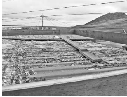
The old, decrepit roof was full of holes that allowed water to leak into the plant.
