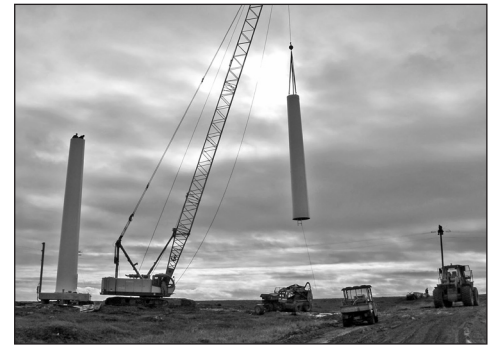
Erecting a wind tower.
