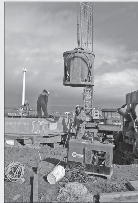
Preparing a tower foundation in Toksook Bay.
