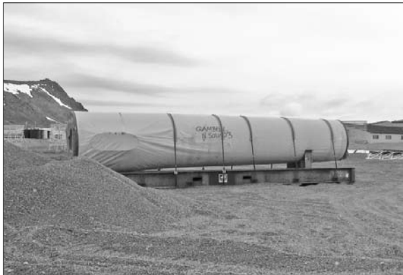
A wind tower section sits at the site, awaiting installation.
