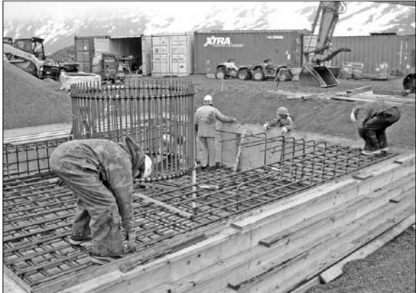
Crews built wind tower foundation platforms out of rebar.
