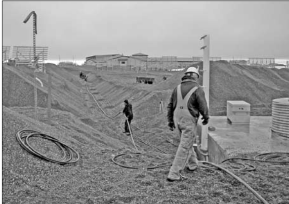
Crews dug a trench to bury the power and communication lines.
