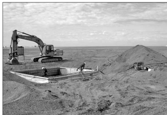
Preparing foundations at Gambell's wind tower site.
