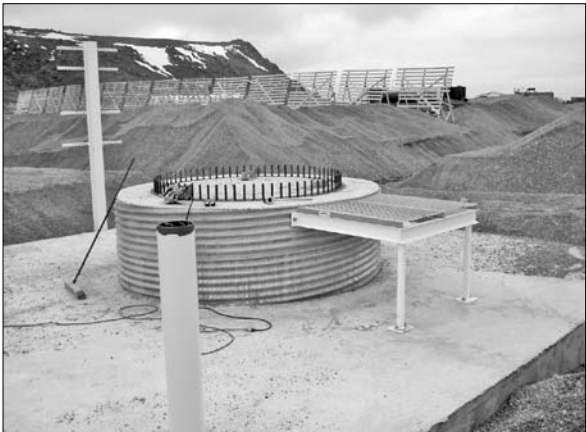
A tower foundation pad after concrete was poured.
