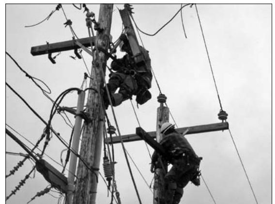
Linemen hooked the wind turbines into a new distribution line.
