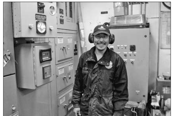
Larry Lake, getting ready to turn off the old control panel.
